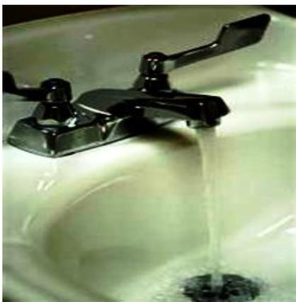
Turn off all of the water faucets or devices once the odor of chlorine has been detected throughout the water system.
