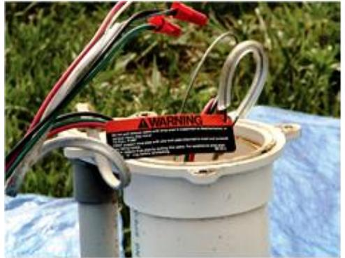
**Pour the 1 gallon of bleach directly into the well casing.** Rinse out the bottle with water and pour that water into the well casing.
