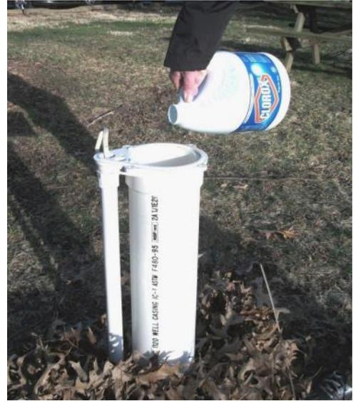
Well disinfection is completed for various reasons and under many different situations, for instance: after work is done on the well casing; when parts like a pump, pressure tank or water line is replaced; or after noticing a change in the taste or smell of the water.
