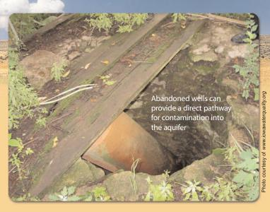
deteriorated to the point that contaminated surface water can infiltrate the well. Abandoned hand-dug wells not only present a contamination concern, they also can create a physical danger to people who can fall into them.
