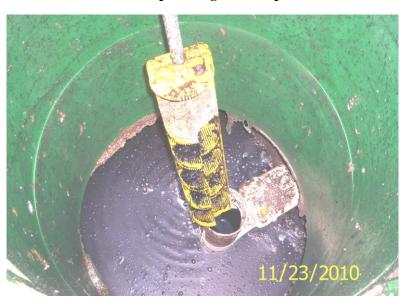
Clean the filter with a hose and spray nozzle. Rinse the solids and waste back into the septic tank.
